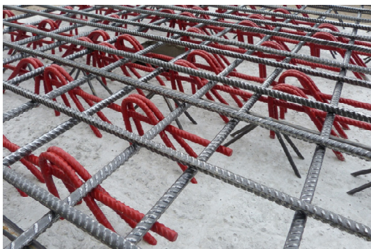
Fig 6 FILIGRAN – Punching Shear Reinforcement with bending reinforcement in place
