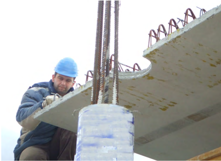
Figure 1: Precast slabs with lattice girders used for composite flat slabs
